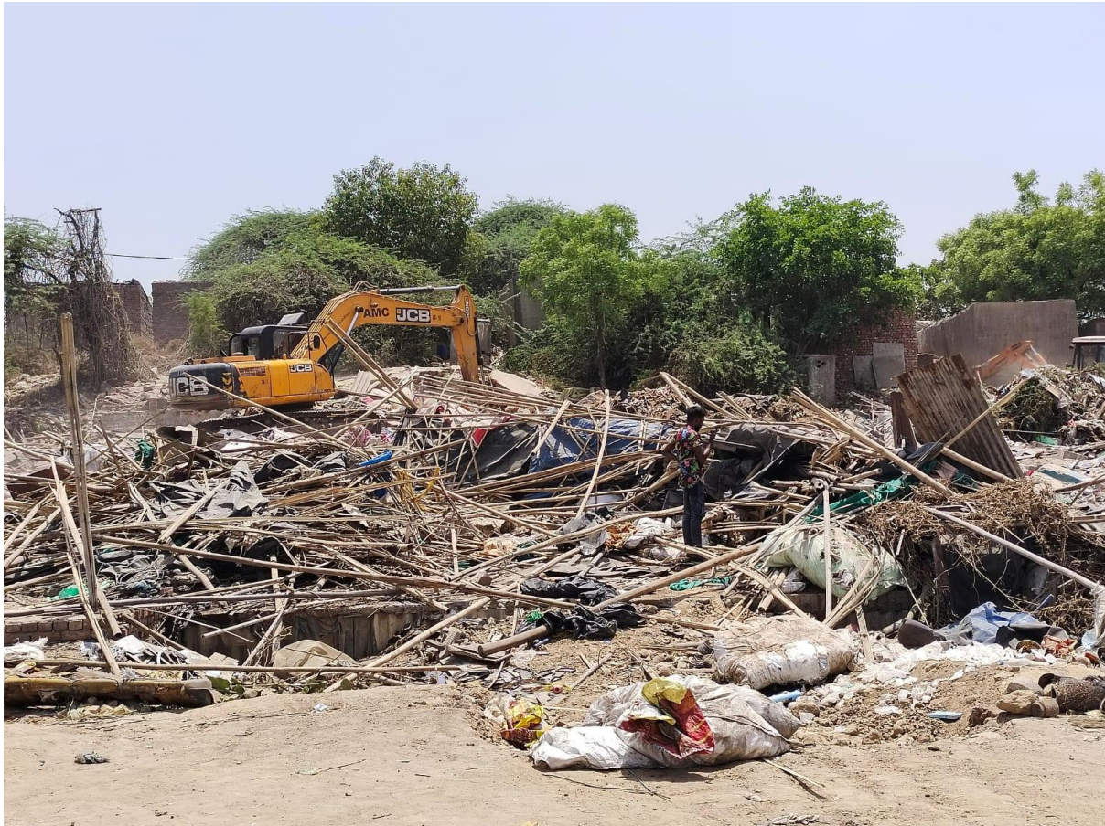
Figure 9: The demolitions in process at Chandola Lake. Photo Credits: Hozefa Ujjaini.
