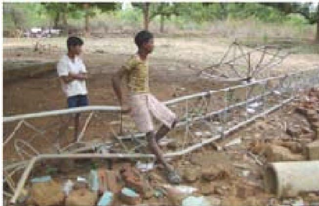
A demolished TV reception tower.
