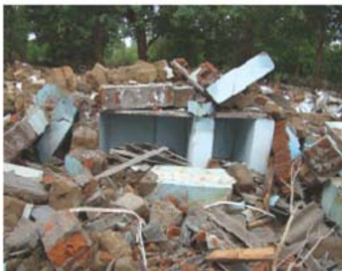
A demolished kitchen and residence used to accommodate participants to various programmes conducted by the VCA.
